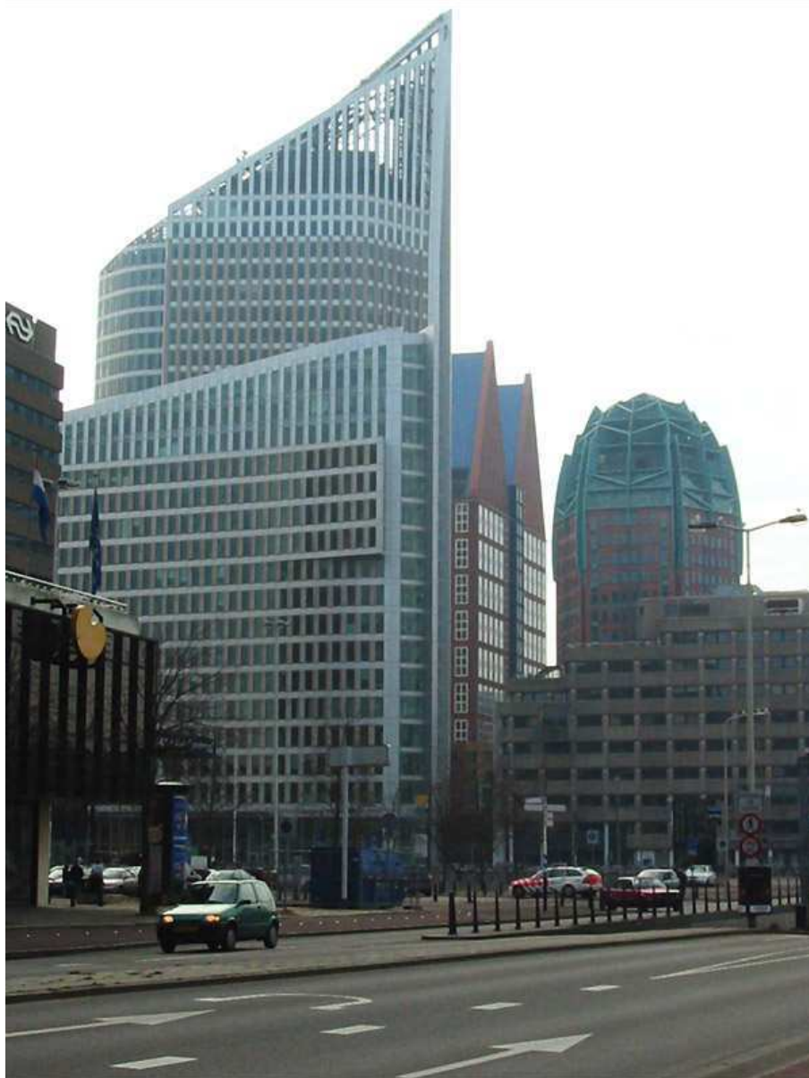
Figure 29: The Ministry of Education, Culture & Science is located in the 'Hoftoren' near the Central Railway station in the Hague.
