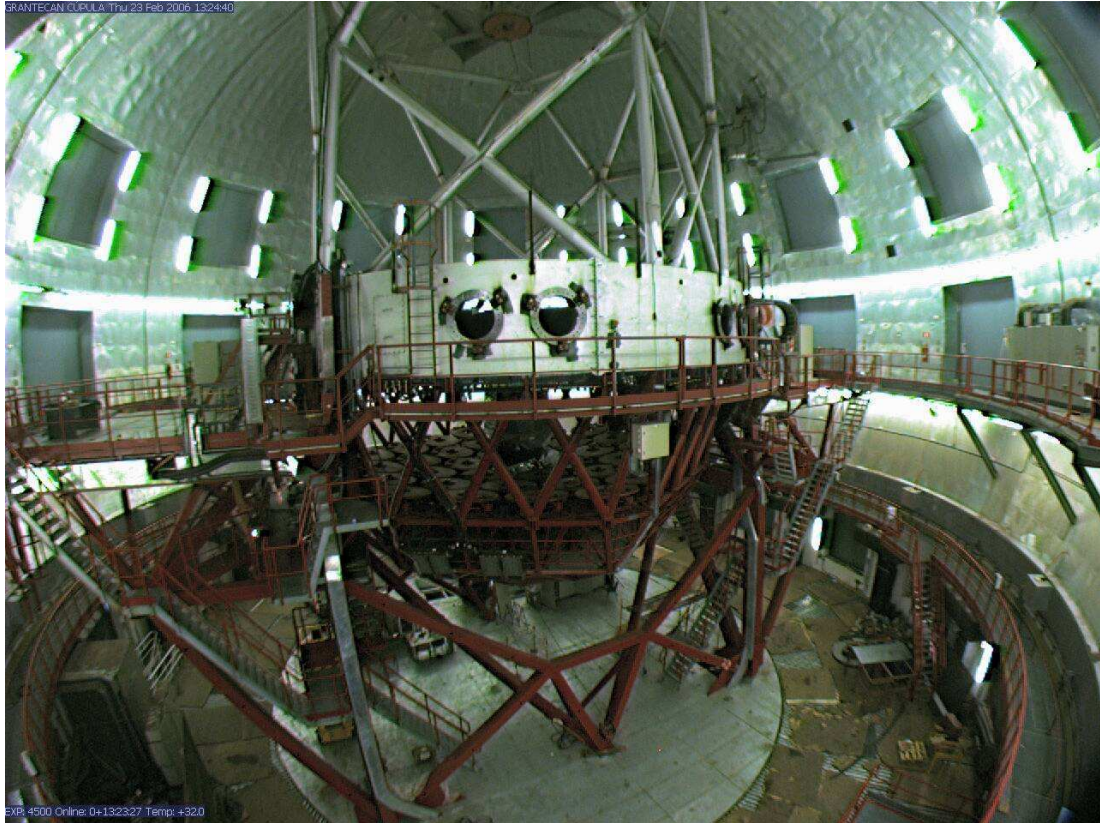
Figure 33: The GTC on La Palma during construction.
