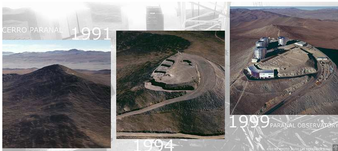
Figure 6: The progress in the building of the Very Large Telescope at Paranal.
