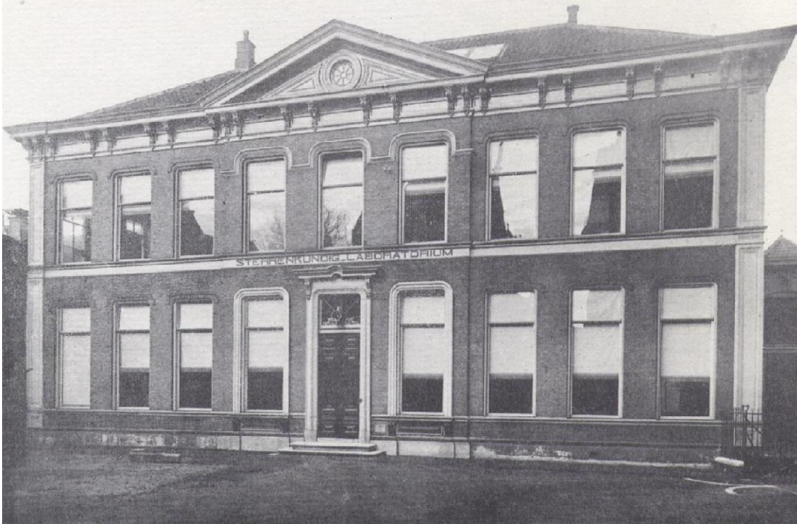
Fig. 4: The building of the Astronomical Laboratory ‘Kapteyn’ in the Broerstraat, slightly to the west of and behind the central university building. The astronomers moved out of it in 1970 and it has been destroyed in a fire in the eighties.
